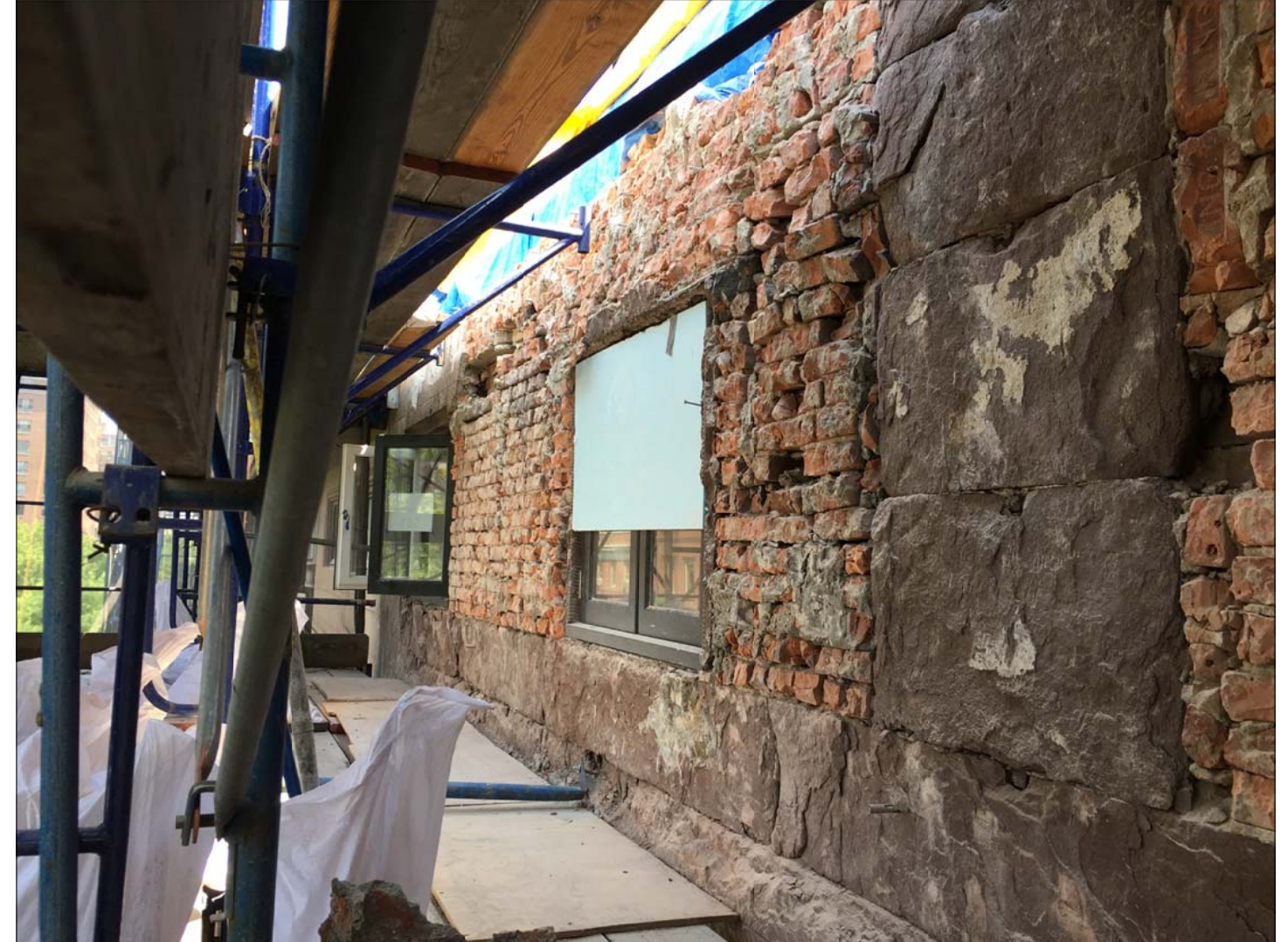
5TH FLOOR EXISTING BROWNSTONE BETWEEN NO. 36 & NO. 38
