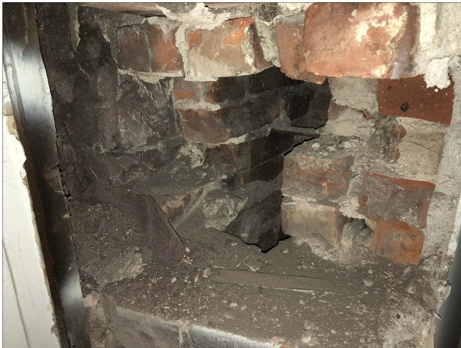
EXISTING FACADE CAVITY WALL AT 38 W10
