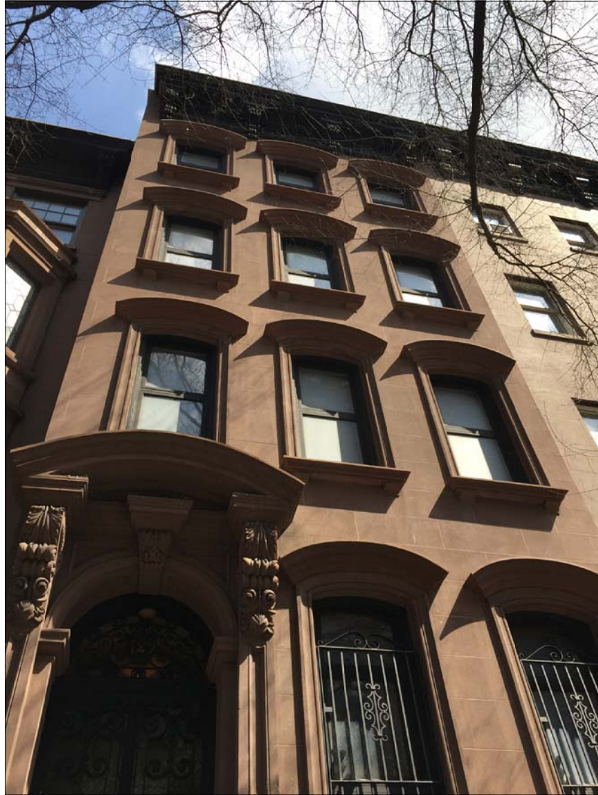
PHOTOS OF COMPLETED FACADE REPLACEMENT AT 129 EAST 35TH STREET UTILIZING CAST STONE MURRAY HILL HISTORIC DISTRICT
