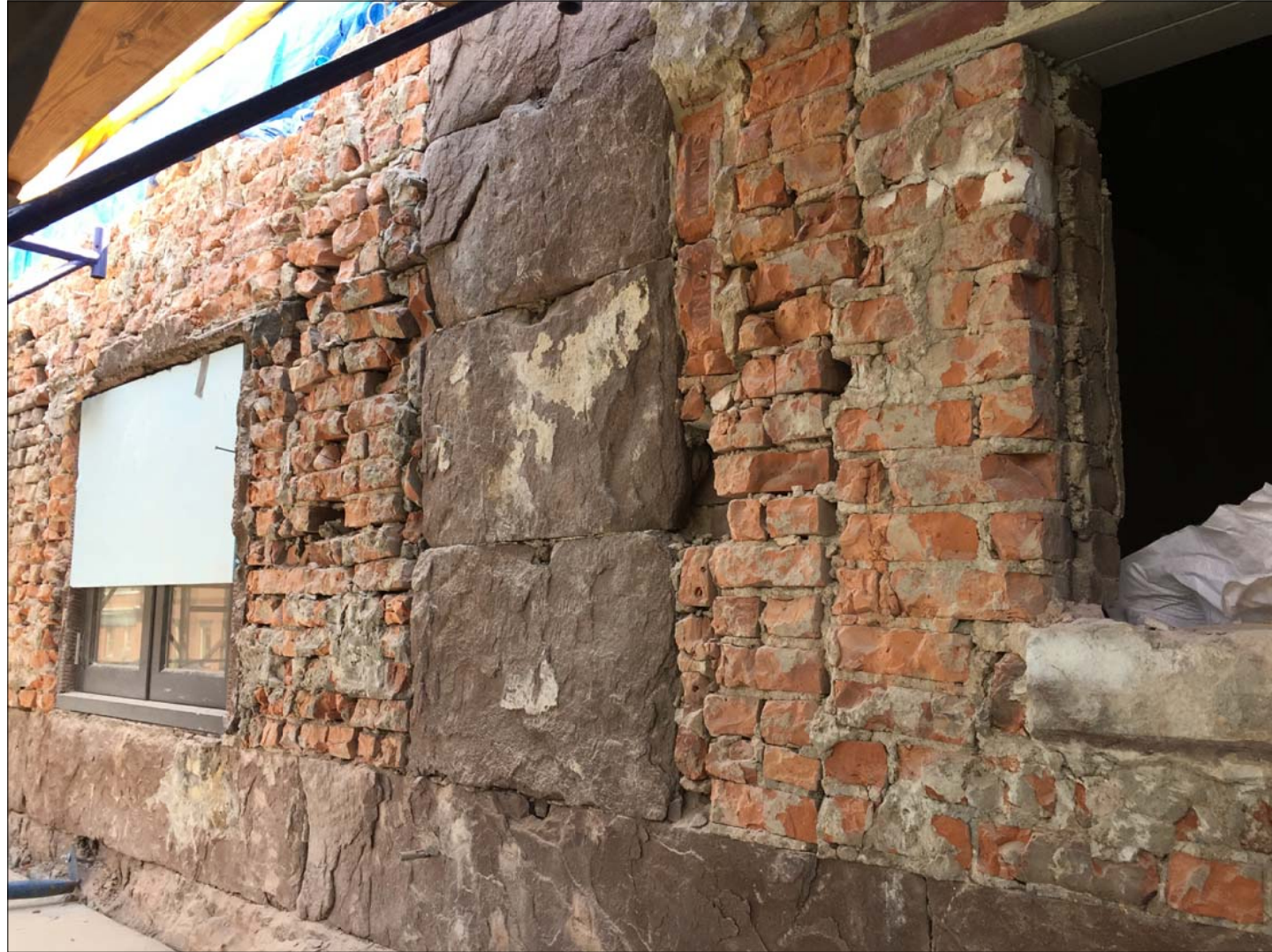
5TH FLOOR EXISTING BROWNSTONE BETWEEN NO. 36 & NO. 38
