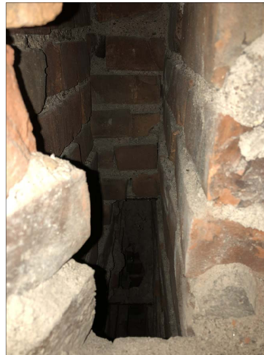
EXISTING FACADE CAVITY WALL AT 36 W10
